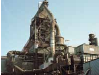
2. Mineral weighing—blast furnace
